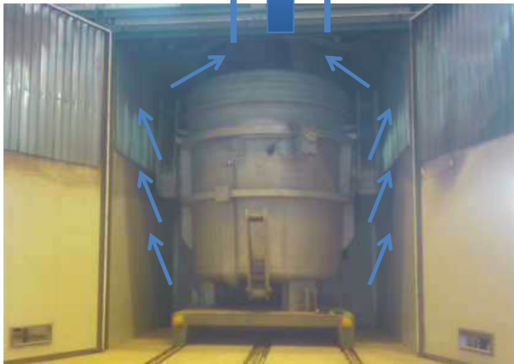
The ladle is closed into a completely sealed box by a dedicated ladle car.
