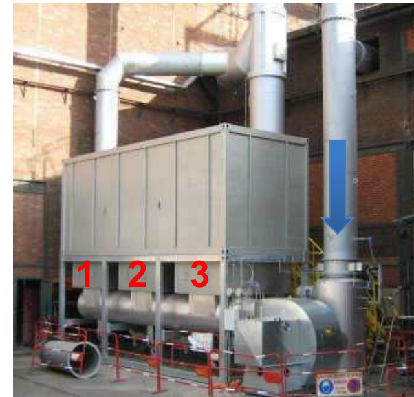
Three regenerative towers with ceramic beds
