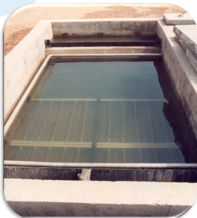
Plates Installed in concrete basin
